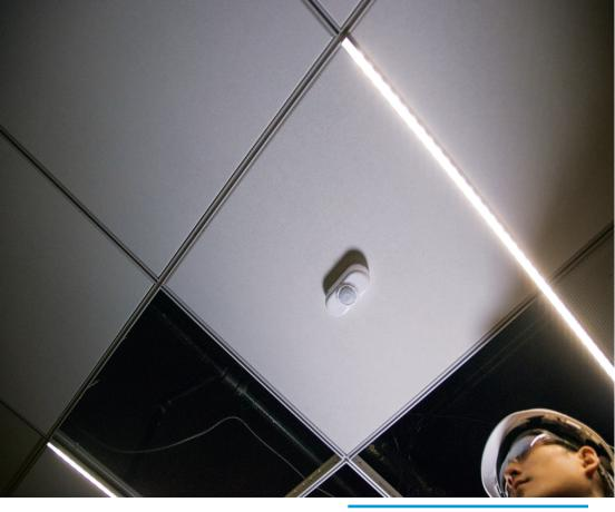
An Audacy Ceiling-Mount Motion Sensor controls the *T-Bar LED*<sup>\*\*</sup> by *JLC-Tech* light fixture in this installation.
